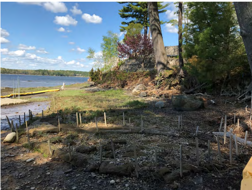
Fig 12: Toe of the slope at Gundalow Landing/east side of the bay. Viewing northwest. (05-11-21)
