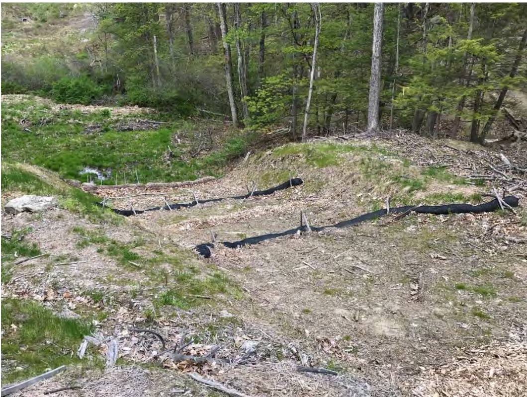
Fig 8: Lower portion of slope between Strs. 28 and 29. Viewing northeast. (05-11-21)
