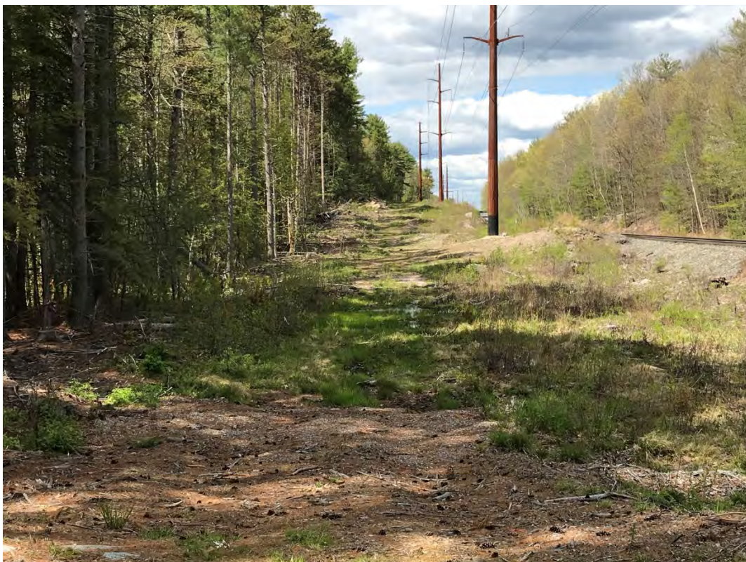
Fig 14: Span between Strs. 15 and 14 containing wetland DW80. Viewing north. (05-11-21)
