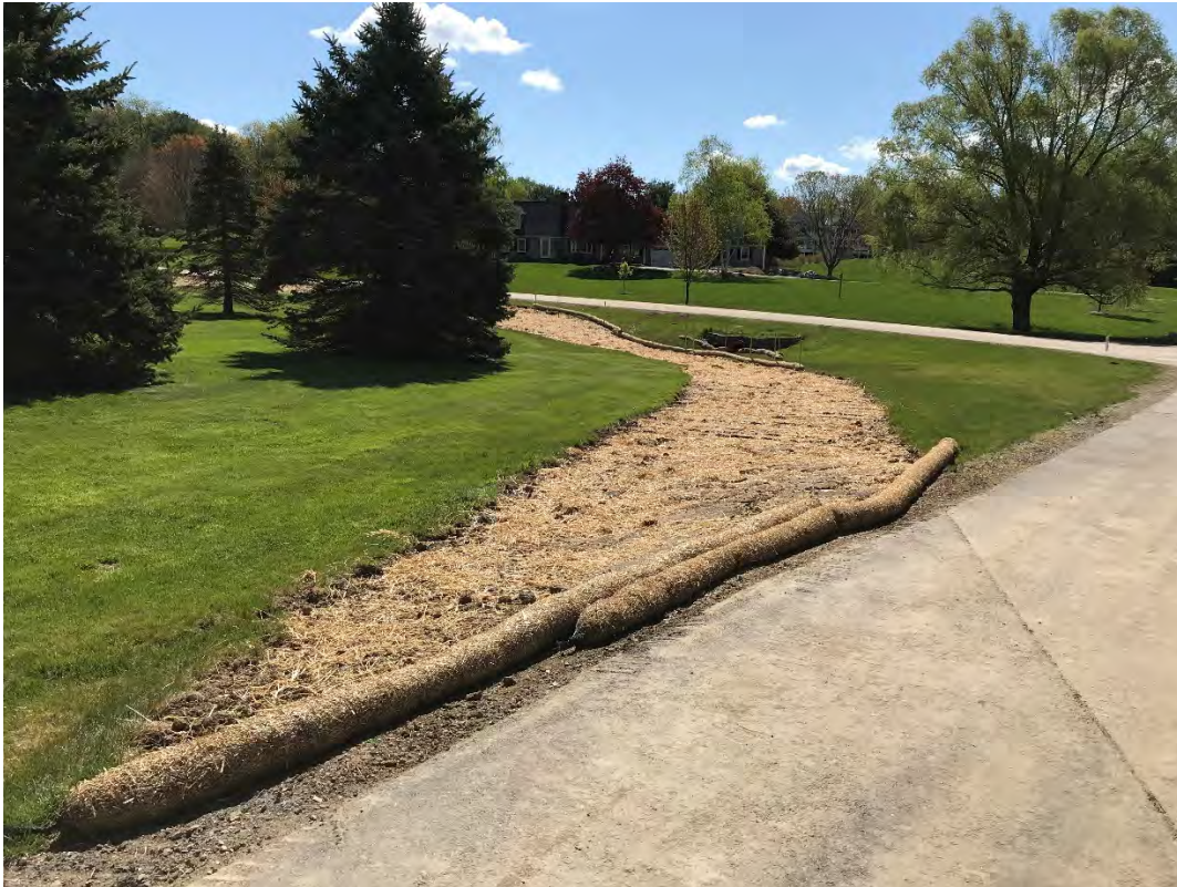
Fig 13: Remediation of flowable fill work site at Gundalow Landing. Viewing southeast. (05-11-21)
