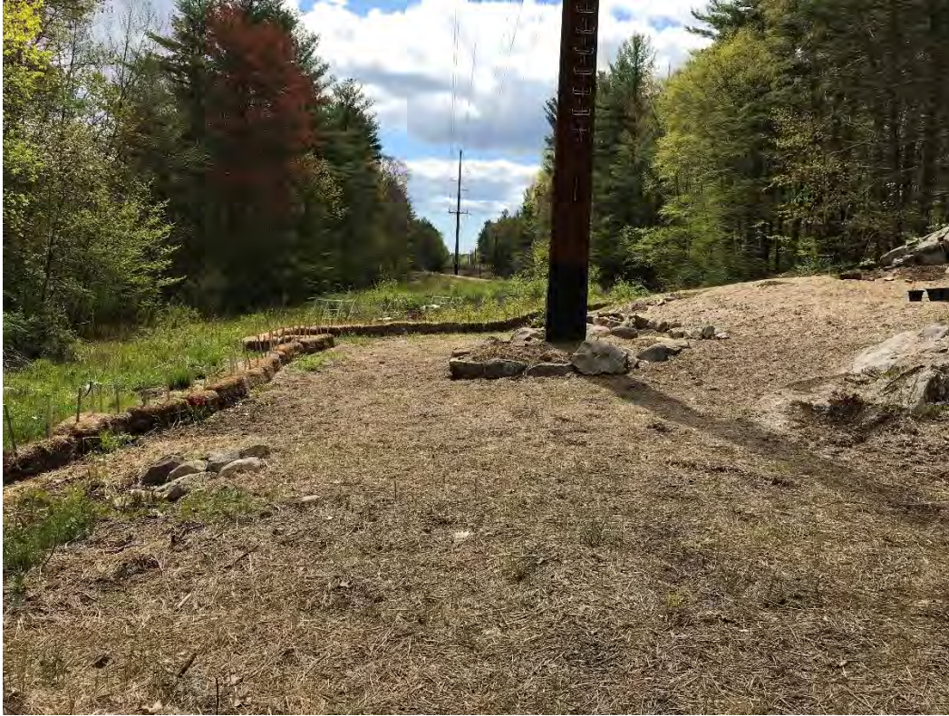
Fig 5: Str. 89 work area. Viewing southeast. (05-11-21)
